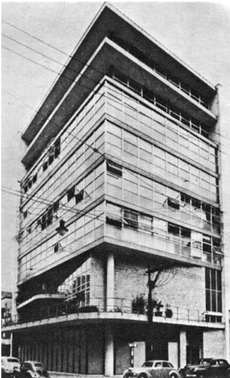
Figure 4 Façade of the Building.
